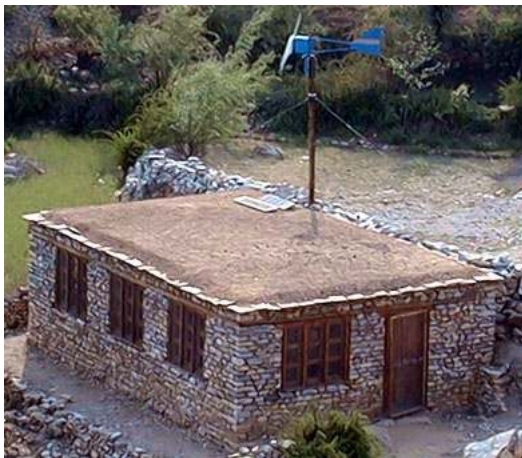
Picture 49: The self made wind turbine charges a 12 VDC battery bank of 150 Ah capacity, enough for one home.
