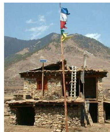
Picture 24: One 40 watt solar PV module for 3 lights
