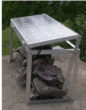
Picture 28: One 75 W R module, adjustable to the season, fixed with stones
