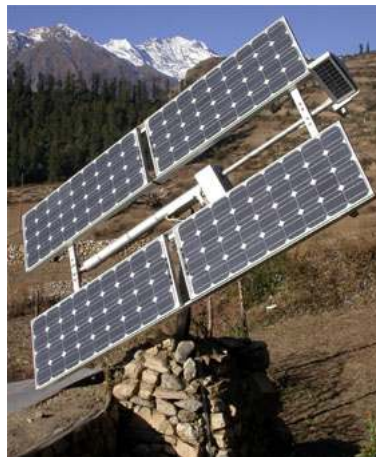
Picture 36: The tracker follows the daily sun path from east-west, and back in the morning to east, by itself.
