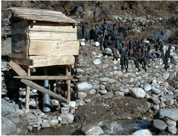
Picture 9: The Thalpi village people built the whole power house and stone/wood water canal, as part of their project input, thus being rightly proud of their pico hydro plant.
