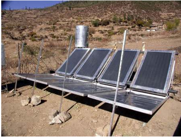
Picture 2: First unit of the Nepali made High Altitude Thermo-Siphon SWH, with opened reflectors, designed to act as night time insulation, beside the ability to empty the absorbers and pipes. A horizontal and 40° fixed angle (same as the absorbers) pyranometer, allow the monitoring and recording of the actually received solar irradiation on the total absorber surface for exact efficiency calculations. The full size (4 units) of the High Altitude SWH bathing center system is designed to provide hot water for 1,100 people, for each to take a shower every two weeks.
