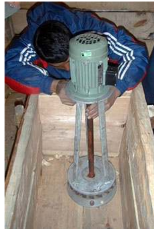
Picture 13: Installation of the Thalpi pico in the wooden canal
