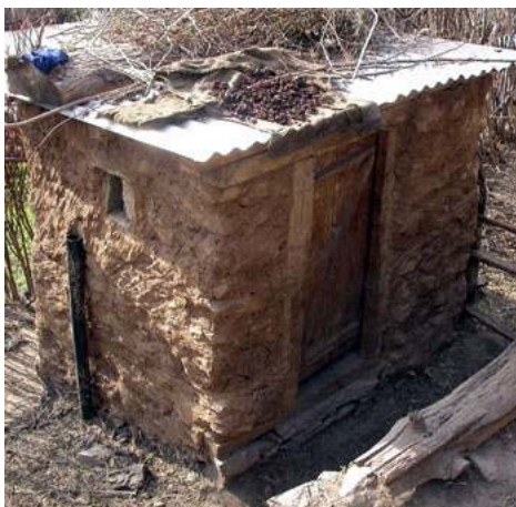
Picture 44: Pit Latrine
