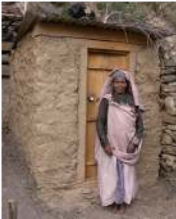
Figure 3-4 Pit latrine for a clean, hygienic environment
