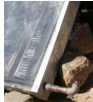
Figure 2-6 Manual water drainage is possible, in addition to the insulated reflector lid. The absorber body is insulated with 50mm glass wool, while the hot water storage tank is insulated with 65mm.
