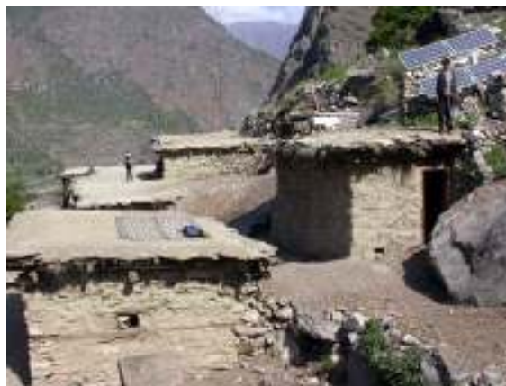
Picture 8: A central village solar PV system with 300 W R for 63 homes and a total of 189 WLEDs for each 5 hours light in each home. That is the Chauganphaya village’s lighting option now since January 2004.
