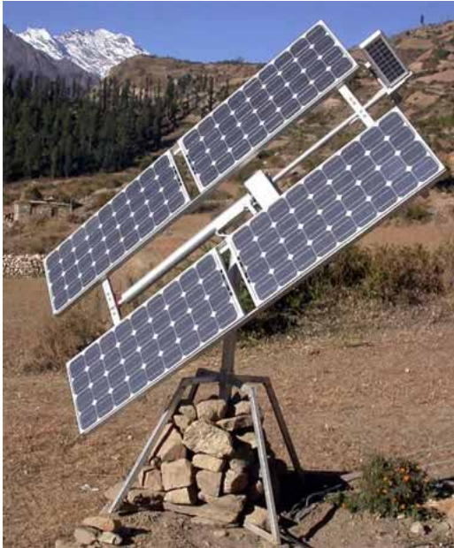
Figure 12-4: 2-Axis Self-Tracking Frame 1 2-axis self-tracking frame for 4 x BP275F solar PV modules. This tracker is installed in the Chauganphaya Village solar PV system.
