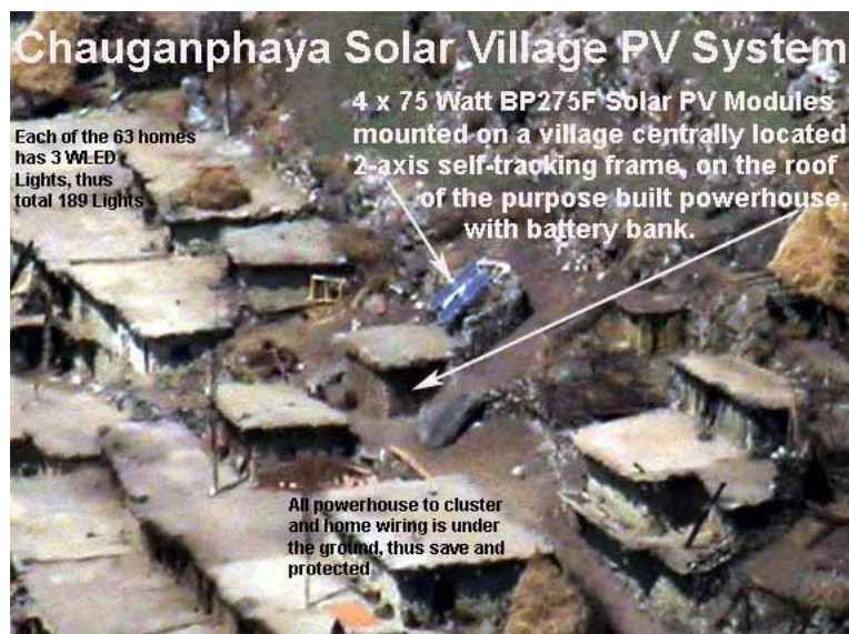
Figure 12-17: Chauganphaya Village Solar PV Power System Chauganphaya Village solar PV 2-axis self-tracking frame and powerhouse. This picture is taken from an air distance of 1.3 km away on the high eastern side of Chauganphaya (see horizon line Figure 9-3, or Appendix 18.8.11. report page 2). As it is typical for this area, people build their homes very close to each other and on top of each other. That saves precious land for their agriculture land, which is their only means to grow food. The various wooden poles seen in the Figure on the flat mud roof tops are not for the transmission line, but are an indication that a shaman (a witch doctor) lives in that home.
