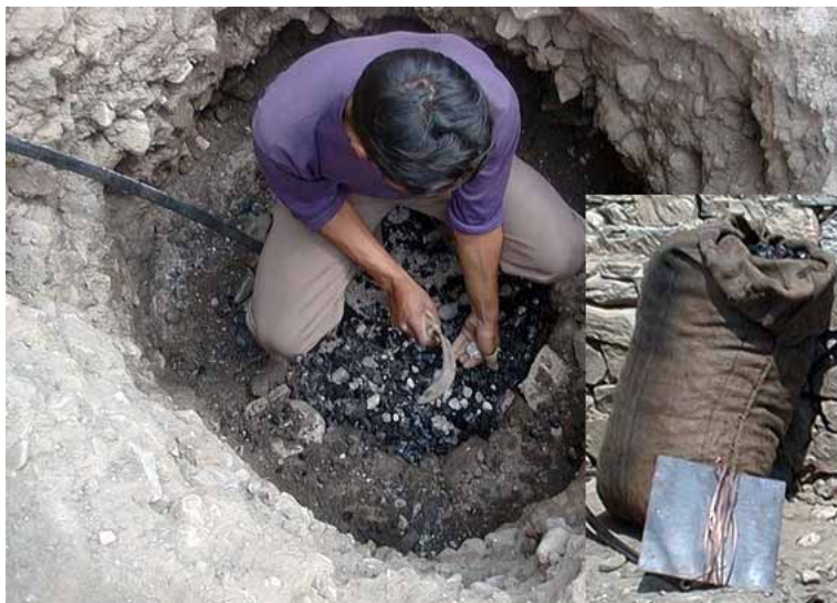
Figure 12-15: Lightning Protection 2 Charcoal mixed with salt provides good conduct.
