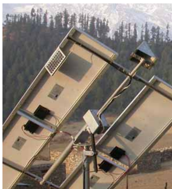
Figure 12-21: 2-Axis Self-Tracking Frame 3 Right after sunrise, the 3 rd 2.5 Watt solar PV module (fixed at the top left of the frame) supports the initial start to move the frame towards East from the fully West position it reached the evening before. On top of the frame in the middle can be seen the two 2.5 Watt solar PV modules mounted with a 30^{\circ} towards each other. One 2.5 W PV panel's plus is connected with the other panel's minus, in order to power the gear box (fixed on the frame) in the direction perpendicular to the sun. In that position the two 2.5 Watt solar PV modules generated equal power and thus the gear box does not turn.
