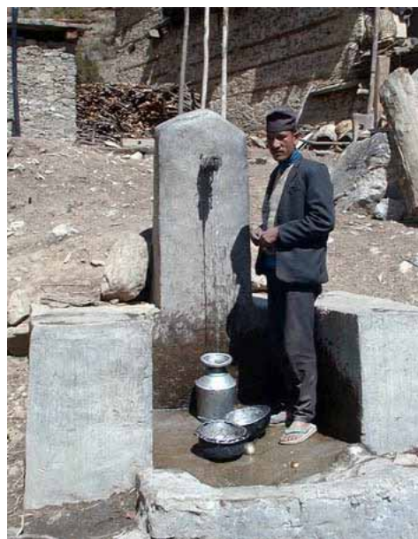
Figure 12-32: Drinking Water Tap Stand 2 The village drinking water systems are all gravity flow systems, with a water spring above the village. That enables a constant water flow, important to keep the system from freezing during the cold 4 winter months from November – February, with temperature down to – 25° C.
