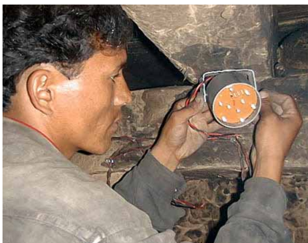
Figure 12-25: Installation WLED Light 2 The installation of the WLED light is important. House wires have to be installed at the bottom or at the side of the wooden beam to protect them from mice. Further the WLED lights are usually installed in the corners of the rooms, under a wooden beam, because they provide a more beam like light and therefore can easier be adjusted under a beam to the place they are intended to brighten up. Further, under the wooden beam they are to some extent protected from the dried up mud, which falls periodically down from the roof.
