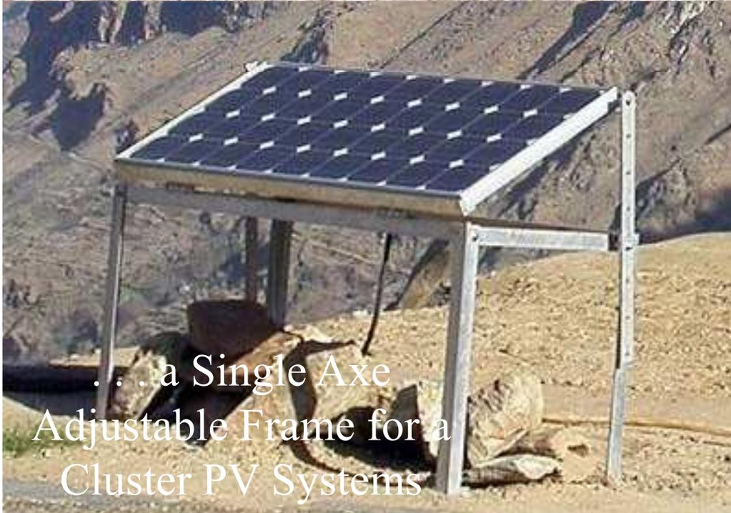
... a Single Axis Adjustable Frame for a Cluster PV Systems
