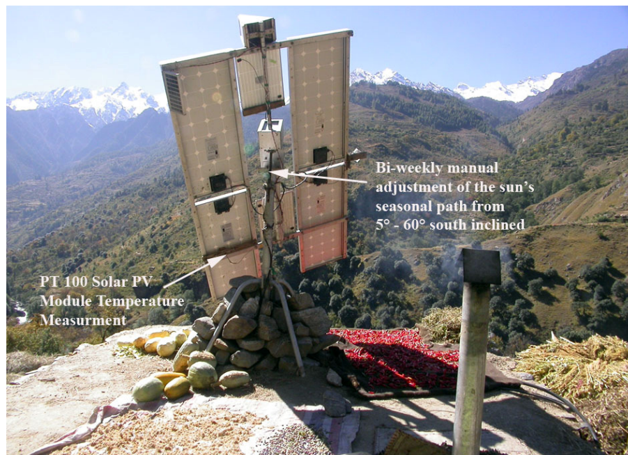
Fig. 7: While the sun's daily East-West path is automatically tracked, the sun's seasonal elevation is bi-weekly manually adjusted. This allows a much simpler technology to be applied for the remote place, increasing the sustainability while minimising the maintenance requirements.
