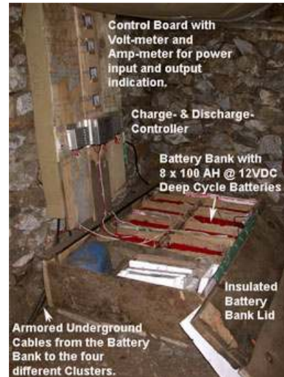
Figure 3-4: Battery Bank well insulated in a locally made wooden box, designed to last 8-10 years, including the load growth.
